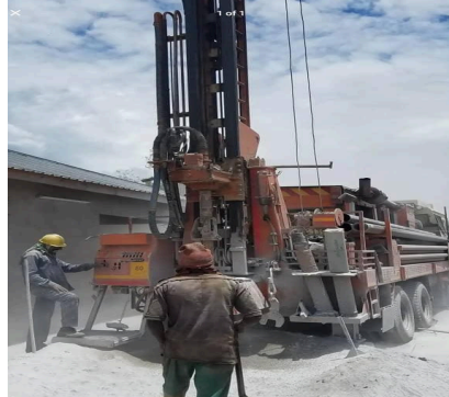
borehole drilling process
