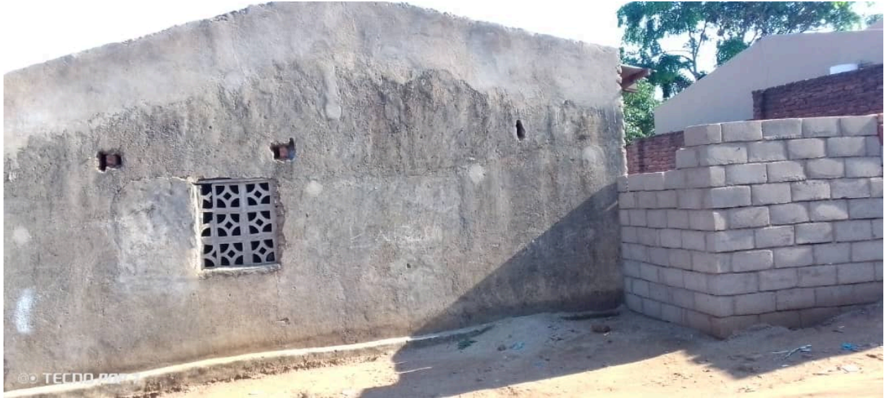
School building left side view
